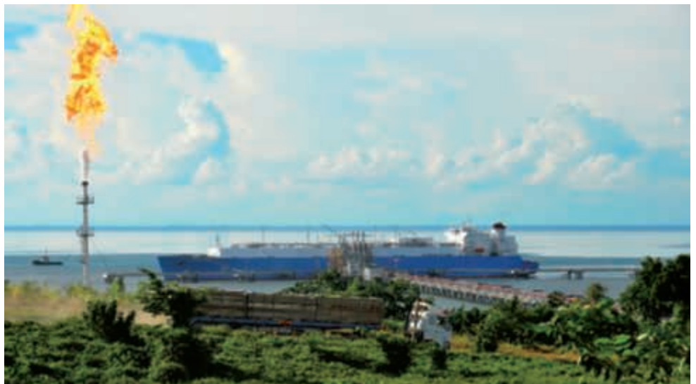
Cegelec in a maintenance contract for BP's LNG plant in Tangguh.
