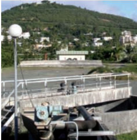
Wastewater treatment plant in Nouméa, New Caledonia
