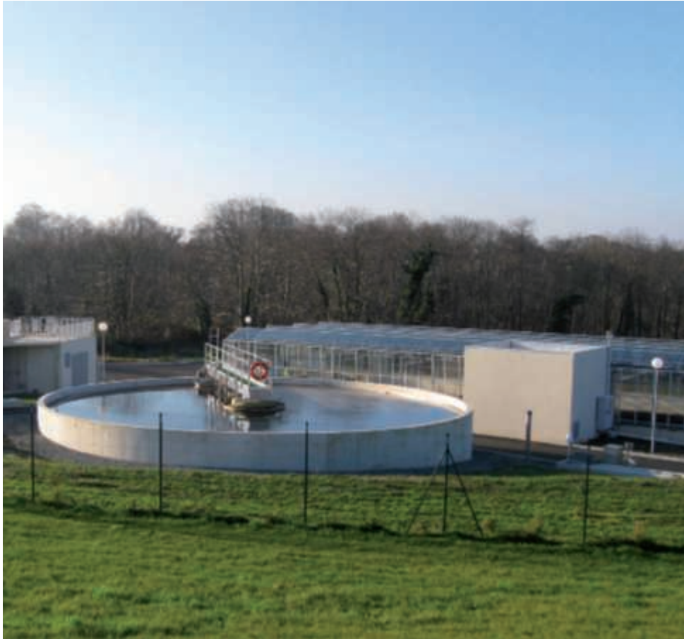
5600 PE wastewater treatment plant with solar drying in Brittany.
